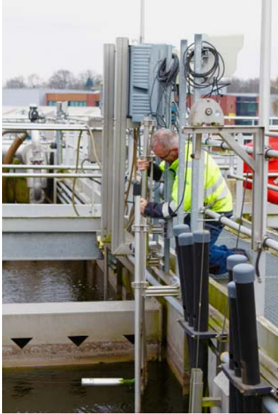
Hach instrumentation at a wastewater treatment plant that uses Nereda® technology
